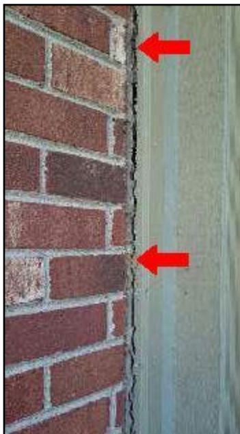
3. Caulking missing or ineffective
