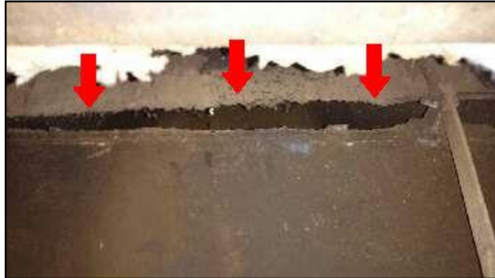
26. Damper or frame rusted
