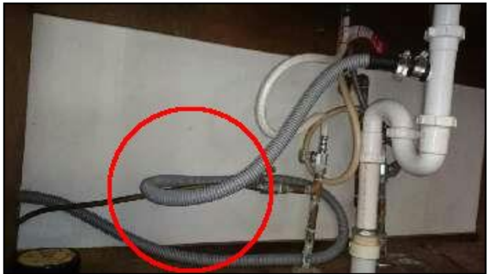
41. Backflow prevention missing
