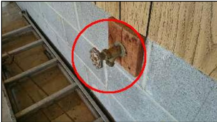
37. Backflow prevention missing
