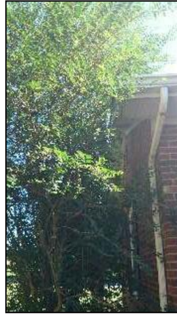
14. Trees or shrubs too close to building
