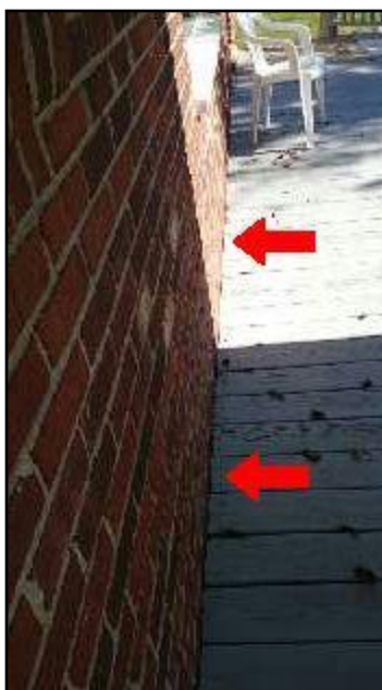
7. Missing flashing at deck connection
