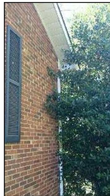
12. Trees or shrubs too close to building
