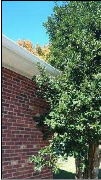
13. Trees or shrubs too close to building
