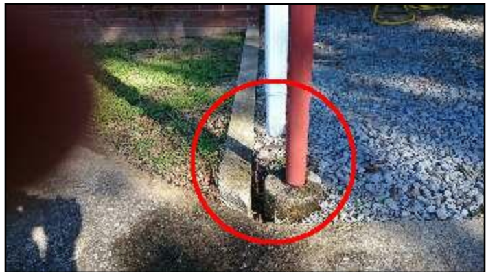
2. Should discharge 6 feet from building
