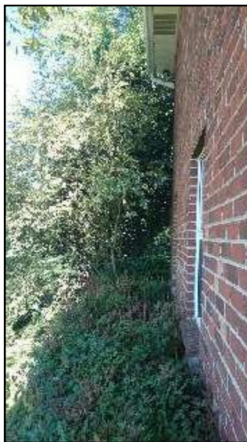
11. Trees or shrubs too close to building
