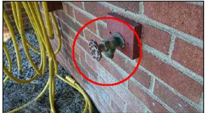
38. Backflow prevention missing
