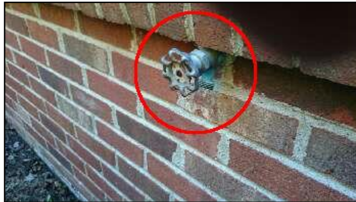
39. Backflow prevention missing
